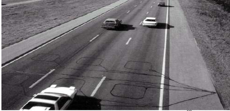
Figure 2: “Inductive Loop Detector System” 69
