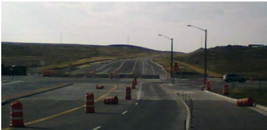
Figure 4: Recent Intersection Infrastructure Construction in Parker 161
